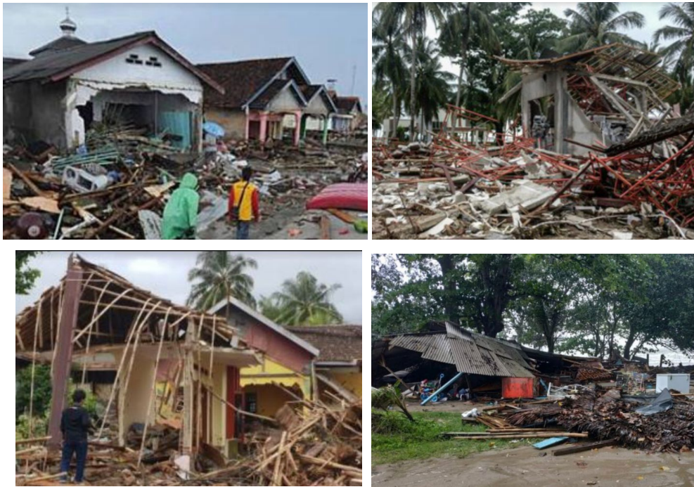
Figure. 3 Examples of poorly built houses from the Selat Sunda Earthquake and Tsunami in December 22, 2018
